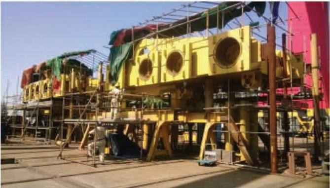
**On-site Milling and Boring of Traveling Cradle**
