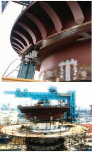
**On-site Machining of Turret Shaft and Caisson**
