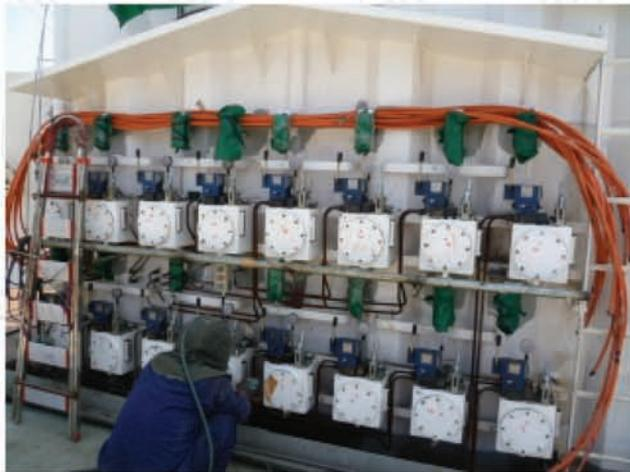
**On-board installation and testing of hydraulic controlled system**
